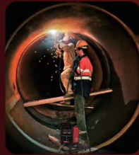
Pipeline Welding
